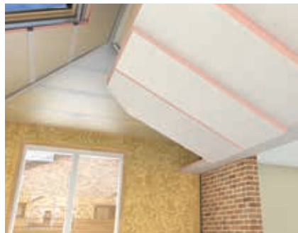
3 layers of high performance insulation (between and over rafters, and insulated plasterboard), is installed.
