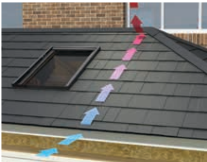
Roof is battened and chosen tile is added ensuring weathertightness. The gutter and external trim are secured.
