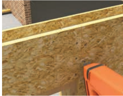
Wall panels are securely fixed together with a nail gun.
