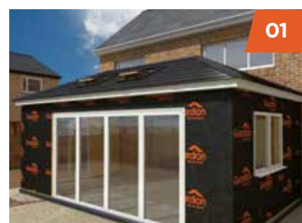
01 Breathable waterproof membrane is secured to the exterior walls.
