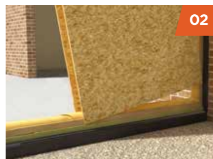
02 Wall and sole plates installed ready to receive the SIP panels.
