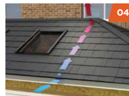
04 Roof is batted and chosen tile is added ensuring weather-tightness. The gutter and external trim are secured.
