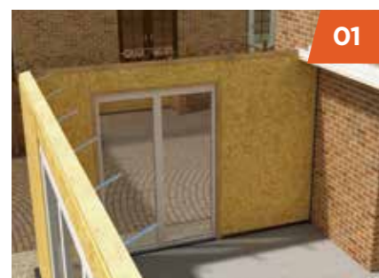
01 Structural ringbeam is sealed and secured to the top of the wall structure.
