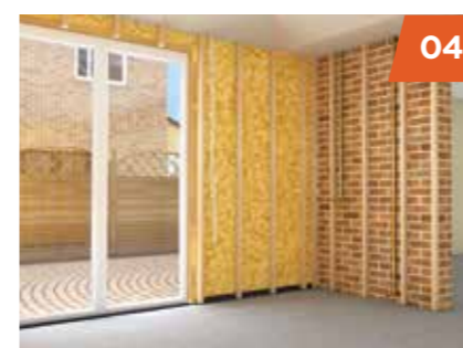
04 The interior has services added and is batted ready for internal finish.
