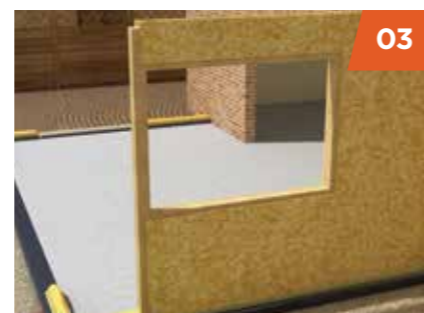
03 Subsequent panels are installed with specified window and door openings.
